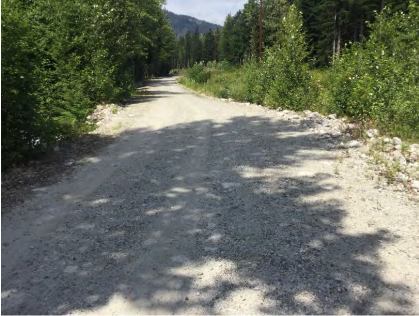
Left Approach Looking Towards Culvert
