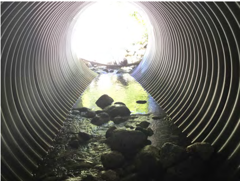
Typical Culvert Barrel Condition
