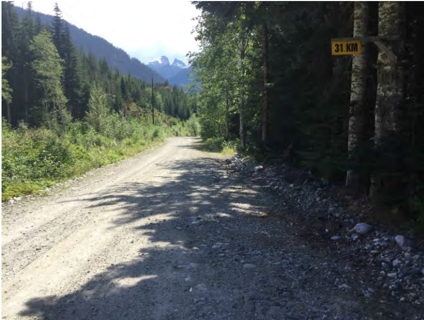
Right Approach Looking Towards Culvert - Note km
