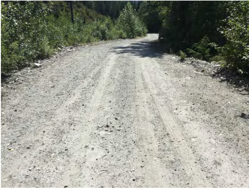
Roadway Over Culvert
