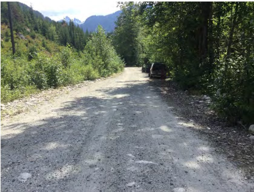
Left Approach Looking Away from Culvert
